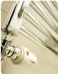
Your radiators may be fitted with Thermostatic Radiator Valves (TRV's). These will adjust the amount of heat emitted from the radiator, dependent on the demand. Each valve can be adjusted by turning the top of the valve. The higher the number displayed on the valve, the warmer your room will become and the more energy you will use. Check your TRV's to make sure they are not set too high.
