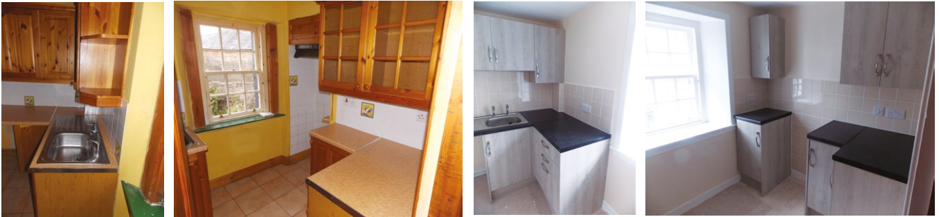
Kitchen improvements (before and after)
