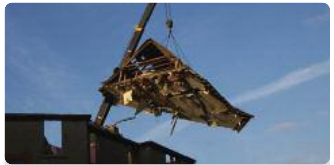
Lifting the roof as part of our demolitions in Campbeltown
