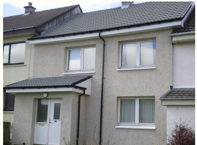
Macdonald Terrace, Lochgilphead - new roof and external insulated render.
