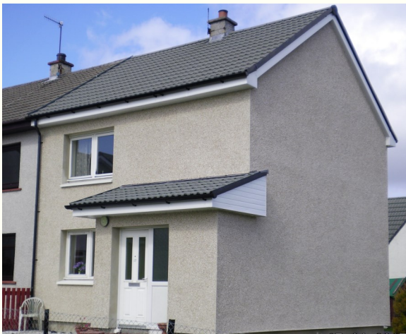
Macdonald Terrace, Lochgilphead - new roof and external insulated render.
